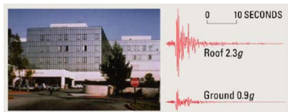
Fig. 3 Amplified signal from floor to roof
